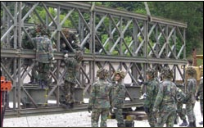
One of the unit's memorable training experiences was constructing a 9-bay double-storey Acrow Panel Bridge at Transit Gap in Nee Soon Camp.
